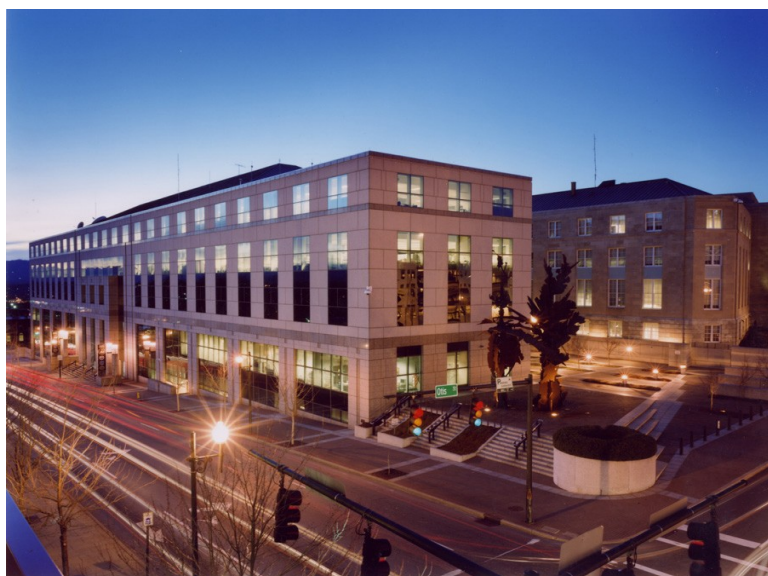
Figure F3: Veach-Baley Federal Complex - NOAA's National Climatic Data Center and CICS-NC
